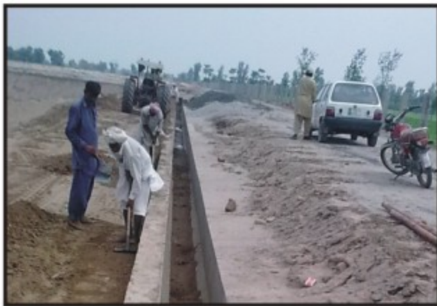
Monitoring visits by PMDFC Engineering Team Landfil site TMACHinot
